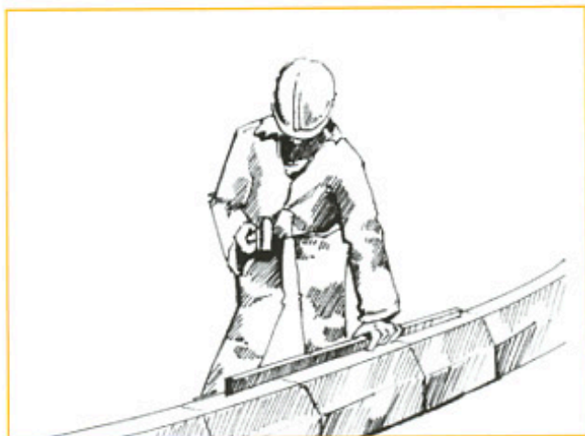
Figure 3: Checking of edge restraints
