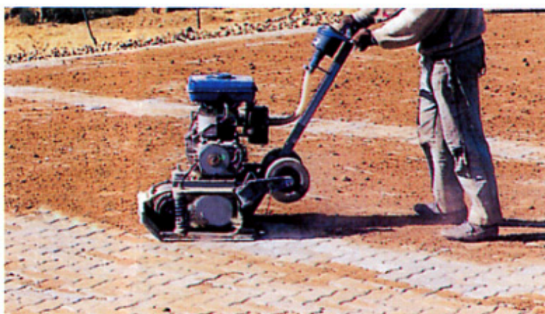
Vibrating the jointing sand into the joints
