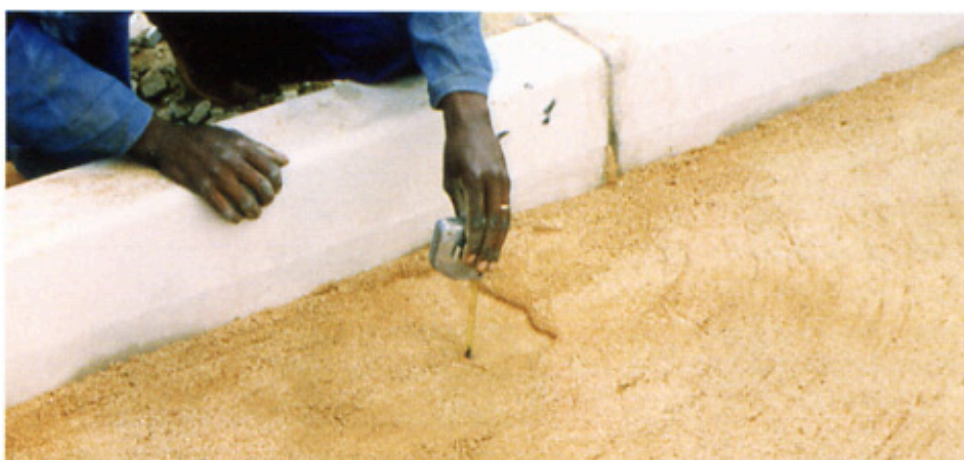
Edge restraints installed before laying commences
