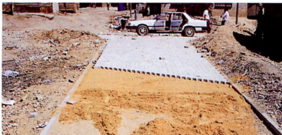
Typical site layout/ construction sequence
