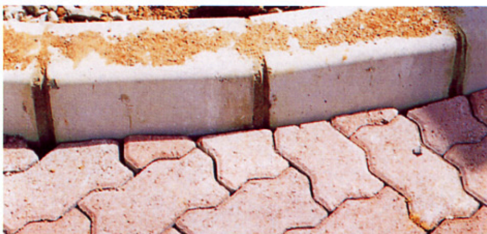
Cutting blocks at edge restraints
