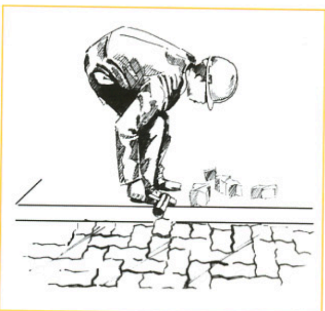
Figure 13: Fitting cut blocks into gaps
