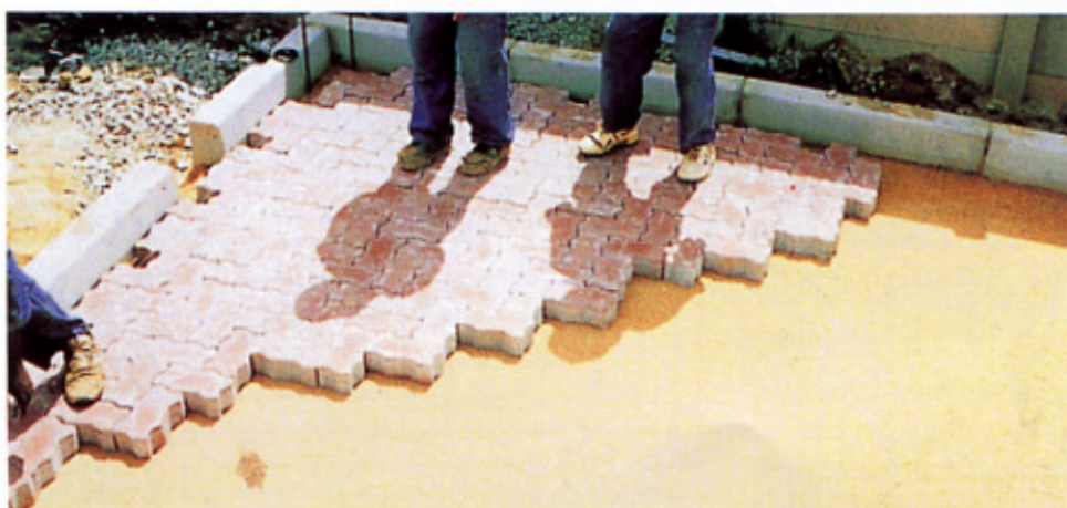
Commencement of laying establishing a diagonal face
