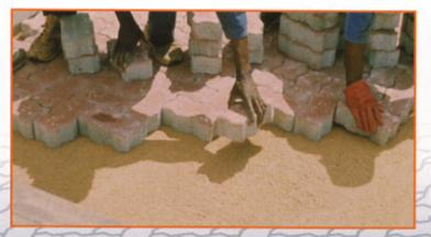
A particularly useful feature of concrete block paving is that it is a 'forgiving' pavement. Thus, where design or construction defects occur locally (such as at manholes, etc.) repairs are not usually difficult, time consuming or costly. Segmented paving also permits easy access to underground services since the paving blocks in the area may be removed. The required work can then be undertaken and the same blocks replaced.
