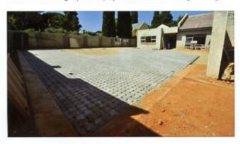
techniques in a sequence, is known as a management train. PCBP manages surface water by attenuation and filtration with the aim of replicating, as closely as possible, the natural drainage from a site before development. The three pillars of PCBP are to:
