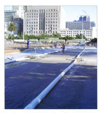
The difference with PCBP is enlarged joints or holes in the corners of the pavers. These joints/holes are subsequently filled with a joint filling material specific to each product, which is an angular aggregate, not sand. This arrangement ensures that water will continue to pass through the joints /holes over the long-term. It is fundamentally unlike pervious materials.
